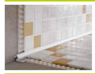
Patented aluminum profiles provide a clean transition between glass mosaic and floor or wall tile. Provideing a hygienic solution to internal corners in kitchen countertops and shower stalls.
